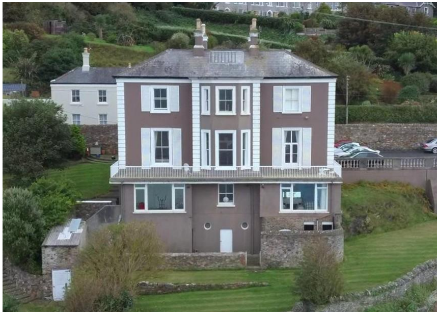
Plate 1: Tara Hall prior to works being carried out
